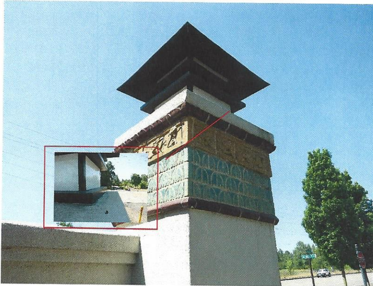
Figure 6 Eastside of Wall Area
