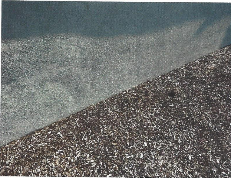
Figure 4 Westside of Wall Area
