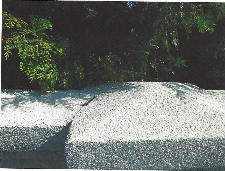
Figure 5 Westside of Wall Area
