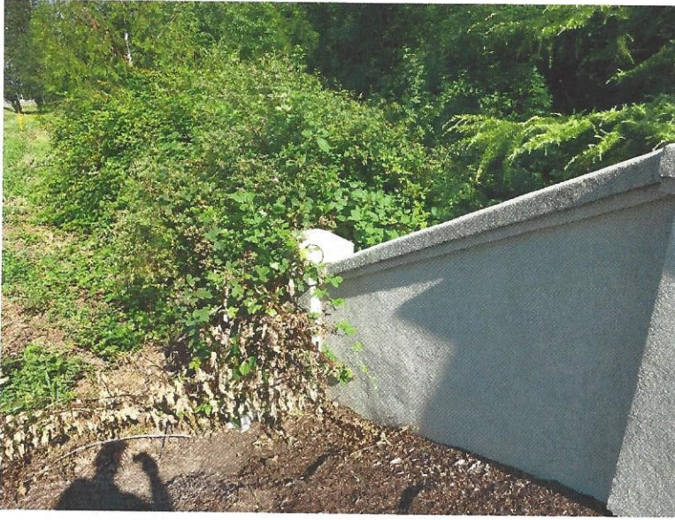
Figure 3 Westside of Wall Area
