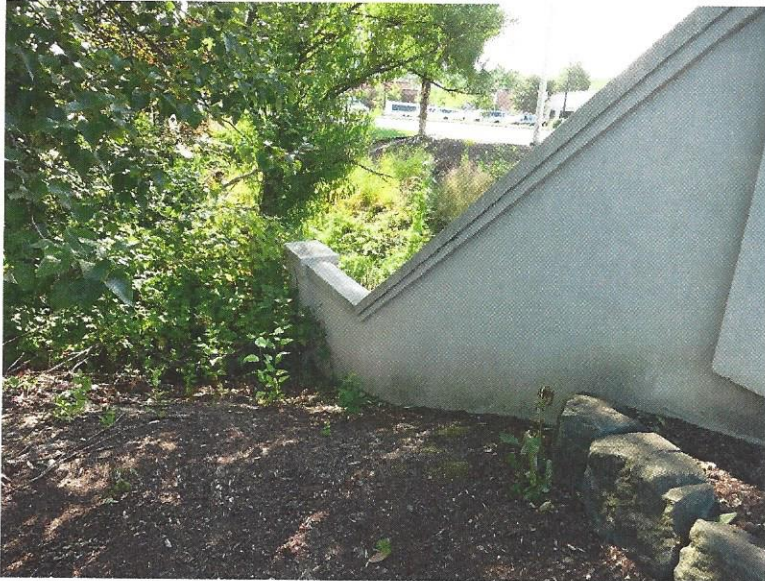
Figure 8 Eastside of Wall Area
