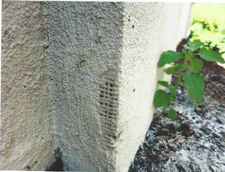
Figure 2 Westside of Wall Area
