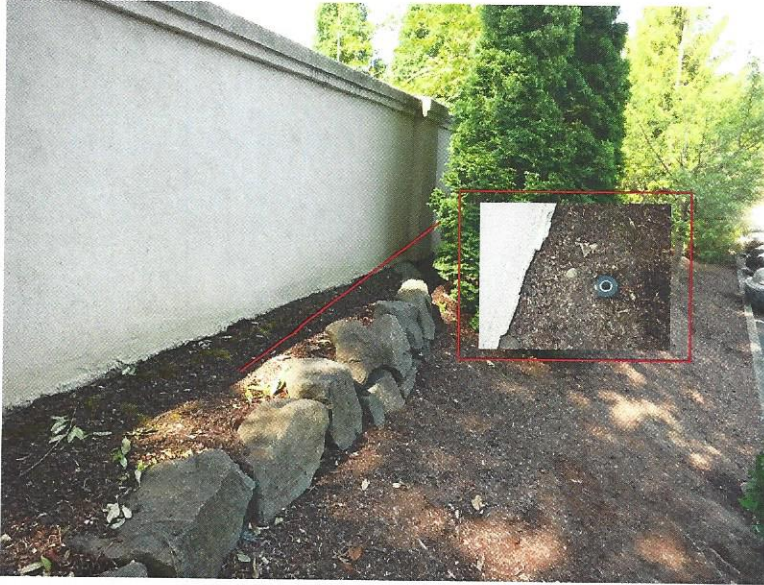
Figure 9 Eastside of Wall Area
